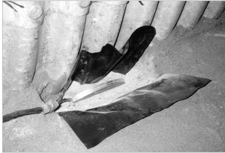
Fig. 6. Earth pressure cell during installation
