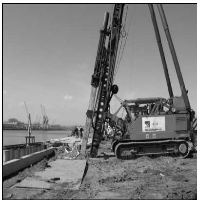
Fig. 3. Driving-in of an inclined pile
