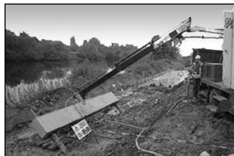
Fig. 4. Static test of an inclined pile
