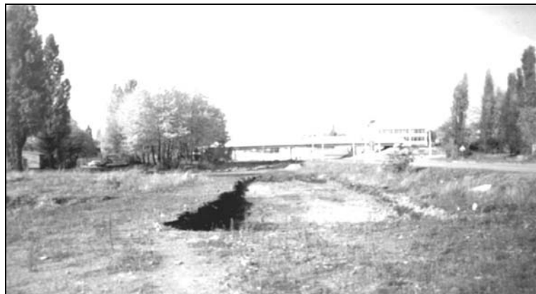
Fig. 20. Example 3. Testing field – shallow excavation in native subsoil
