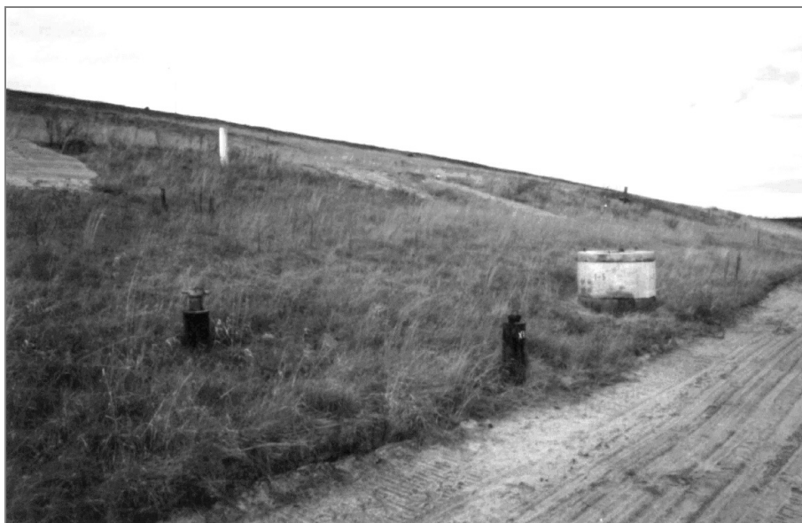
Fig. 3. Benchmarks on the eastern dam
