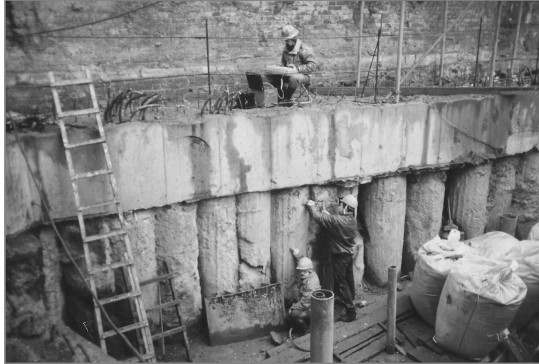
Fig. 6. Conditions of field operations by seismo-acoustic sounding piles
