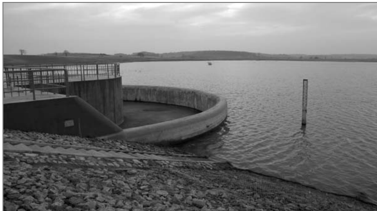
Fig. 3. The view of the dam's frontal overflow crest in normal conditions of water storage
