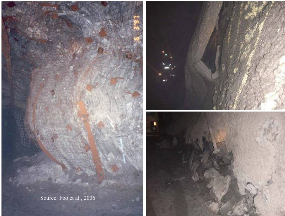
Fig. 17. Effectiveness of bolting and meshing (left) vs. SFRS in controlling ground deformation (top and bottom right)
