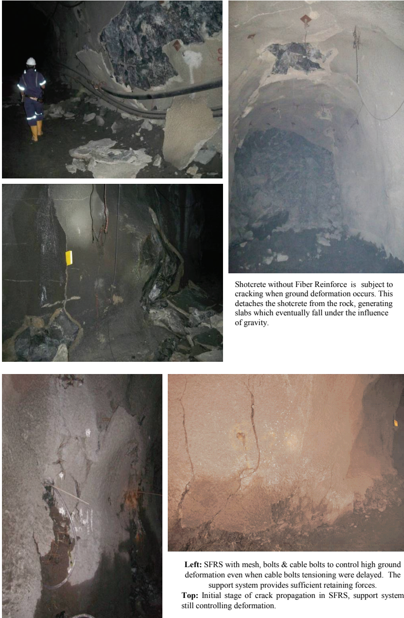
Fig. 13. Examples of shotcrete applications in weak rock mass
