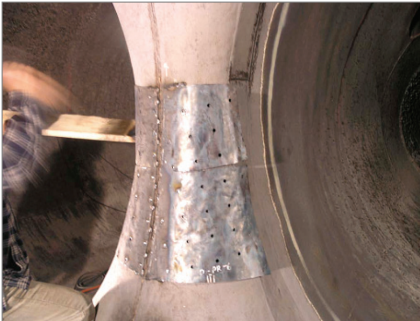
Fig. 16. Quadrangular components of the reinforcement in the process of tacking along centerline of the branch.
