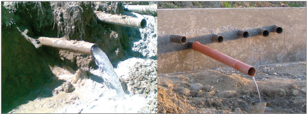
Fig. 3. HDB discharge during drilling and two months after
