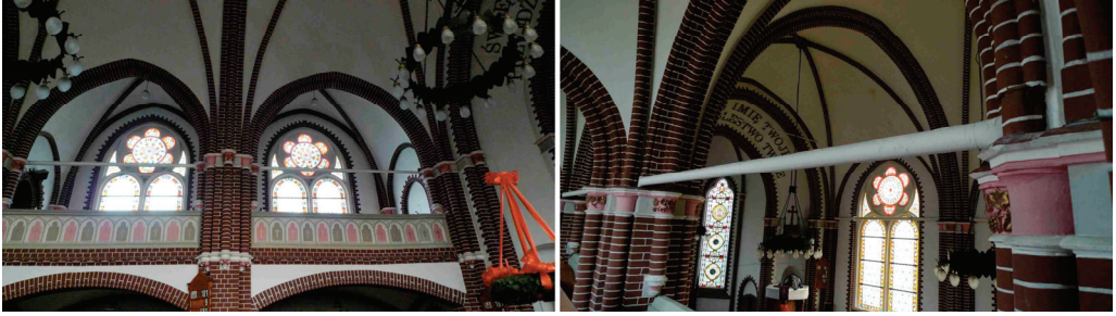
Fig. 4. Steel tie-beams protecting against mining damage
