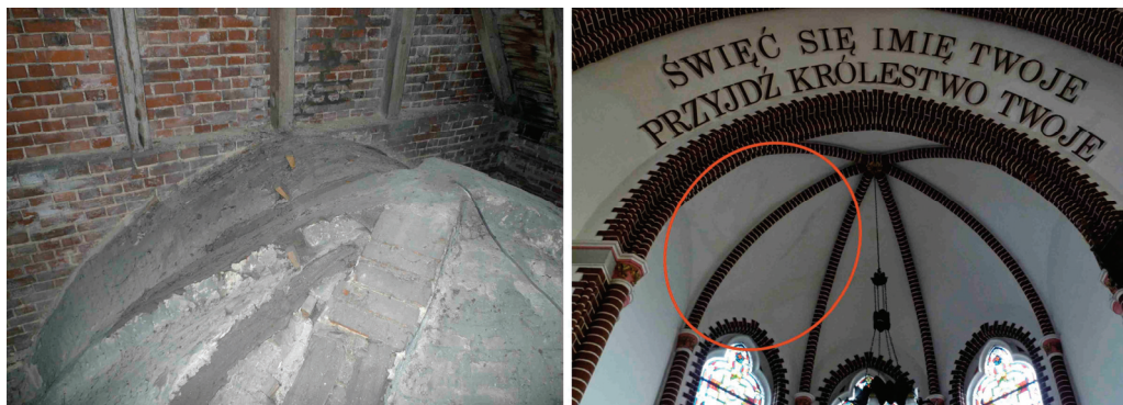
Fig. 8. Repair work done to top and bottom surfaces of vaults
