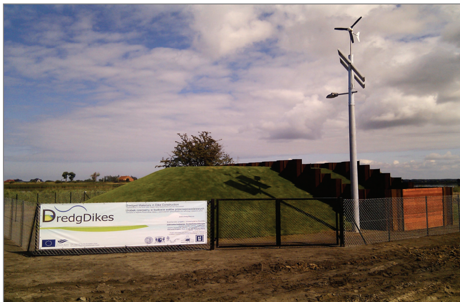
Fig. 1. View of the test dike
