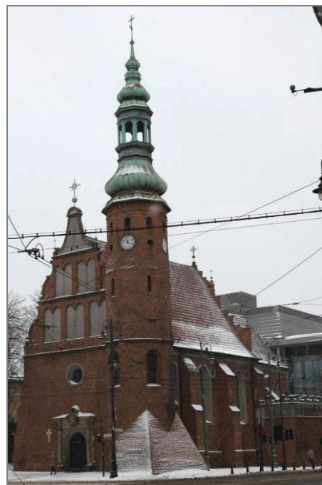
Fig. 1. A general view of the damaged object, March 2013
