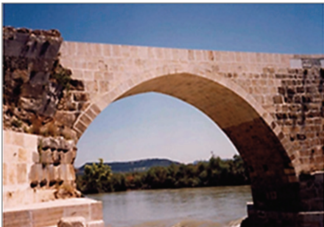
Fig. 1. Present-day use of travertine in the renovation of historical engineering objects – Belkis bridge (Turkey) (photo by J. Pinińska)
