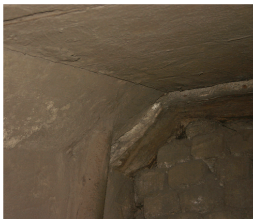
Fig. 2. Vertical displacement on the joint of the L-1 segment of the ventilation duct with shaft collar, from the shaft's side
