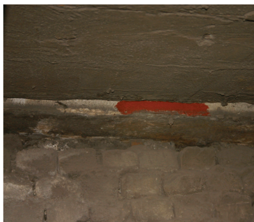
Fig. 2. Vertical displacement on the joint of the L-1 segment of the ventilation duct with shaft collar, from the shaft's side
