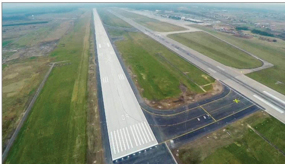
Fig. 1. New runway at the Katowice Airport built in 2014, [16]
