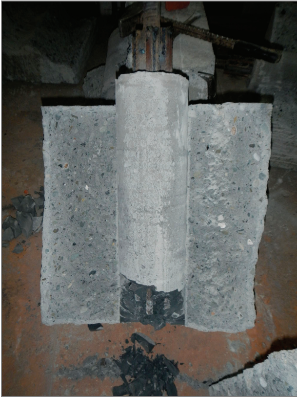
Photo 15. Damaged concrete foundation specimen
