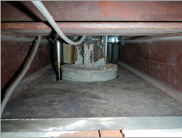
Photo 12b. Displacement of pile head in brick foundation specimen
