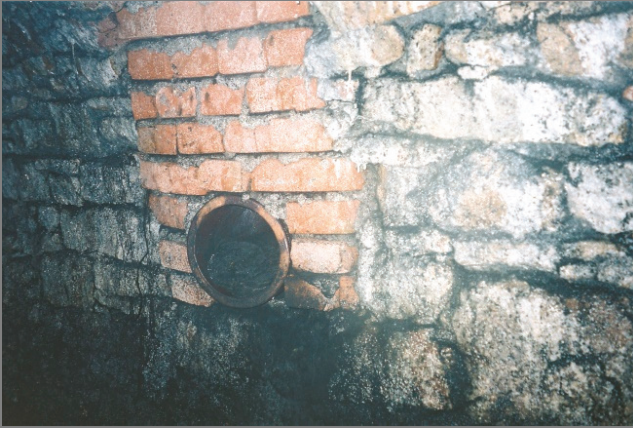
Fig. 4. Sewage connection to the adit (Photo: W. Preidl [14])
