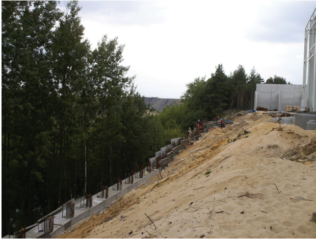
Figure 2: Embedded wall under construction.
