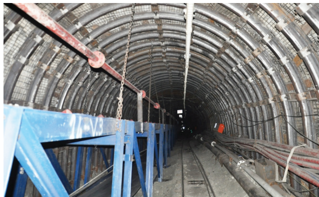
Figure 2: General view of the gallery [11].
