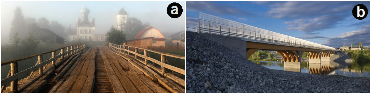
Figure 1: a. Wooden bridge in Kenozero National Park, Russia (Alexey Kudenko/RIA Novosti). b. Wooden bridge (160 m), designed with glulam beams in the Crie de Mistissini, Canada.
