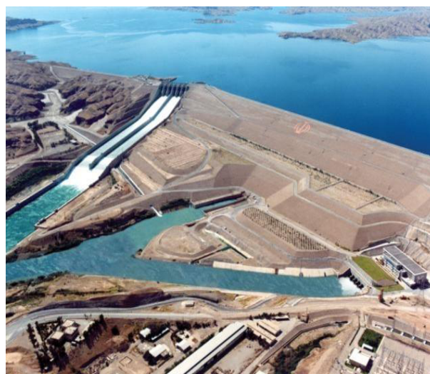
Figure 1: Karkheh Dam, Iran.
