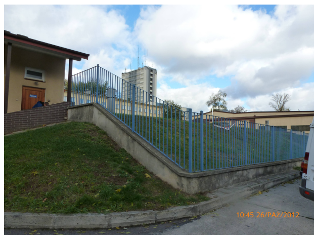
Figure 1: The outside view of water tank.
