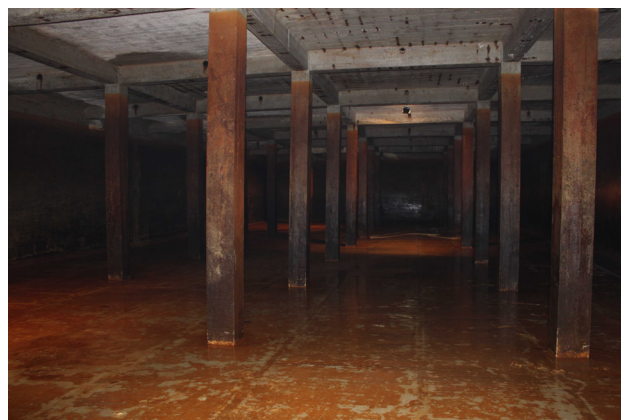
Figure 2: The interior of concrete tank.
