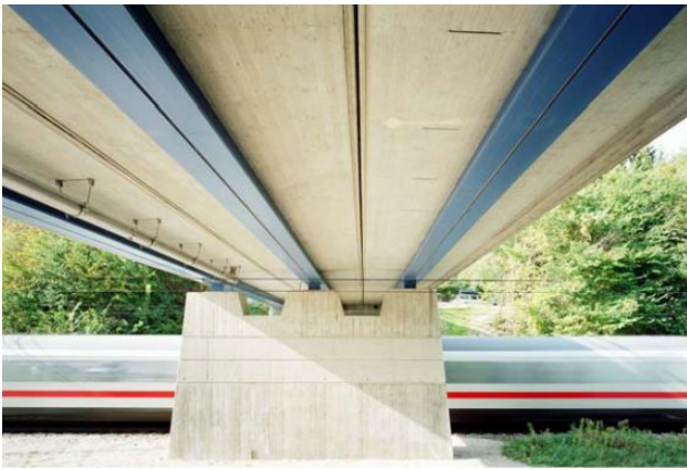
Figure 6: Composite girders of the viaduct in Pöcking [50] with puzzle-shaped dowels.
