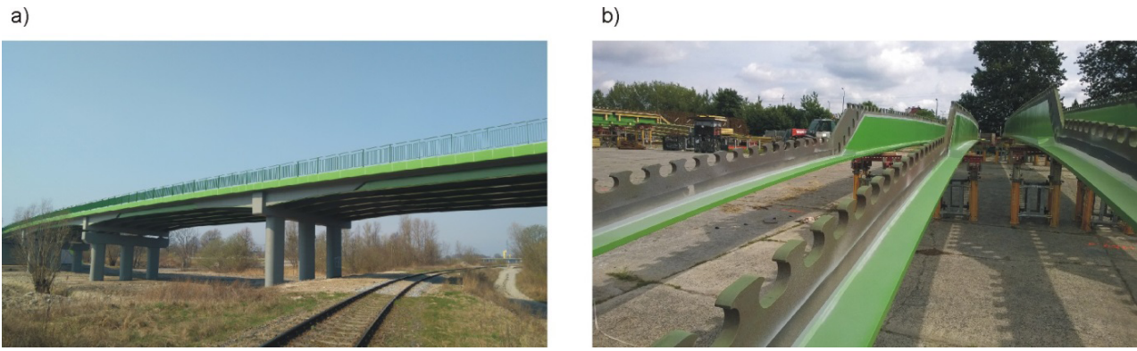
Figure 1: Steel-concrete hybrid beams of innovative composite bridge constructed using composite dowels in Poland, 2016.
