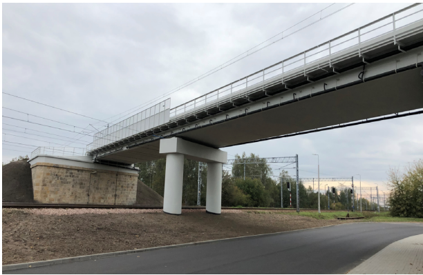
Figure 5: General view of the bridge (picture by Nowak Mosty).
