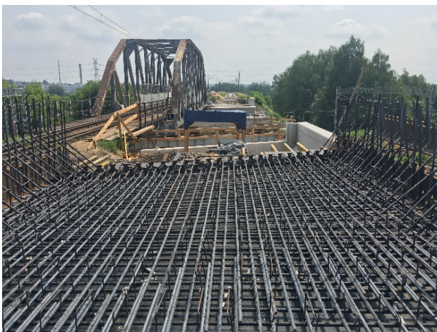
Figure 15: The general view of slab reinforcement.
